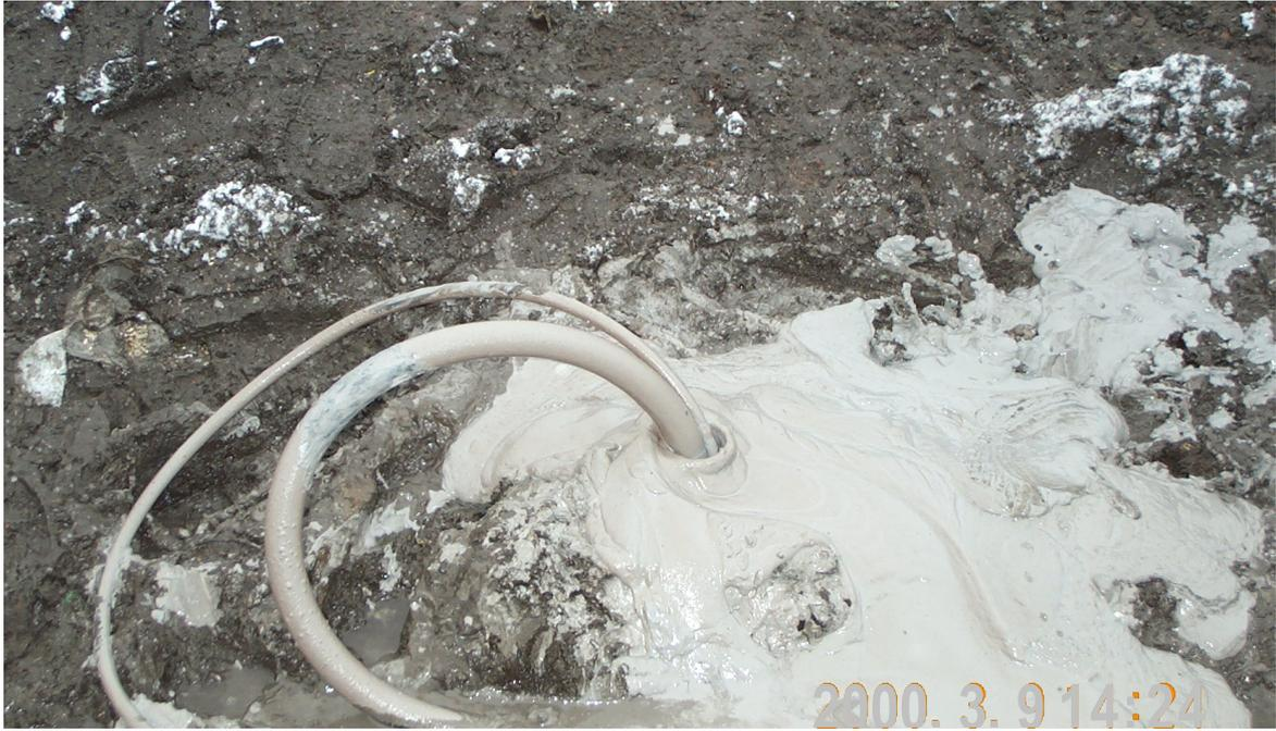
Figure 3. Slurry of fly ash and water around an injection hole with injection hose and hydraulic hose. The slurry rose outside the injection pipe and also inside the pipe after the pressure had been removed from the sleeve.
